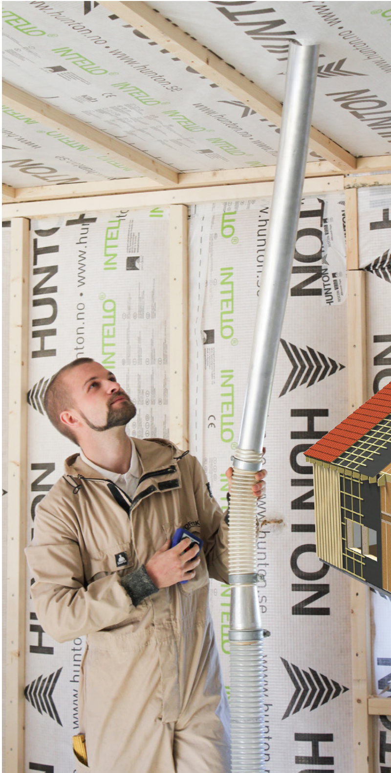
Illustration shows wall insulated with Nativo Wood Fibre Blown-In Insulation.
